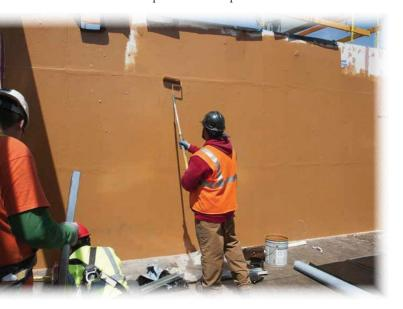
An installer applies Cat 5 primary air and waterproof barrier to GlasRoc sheathing on the ground floor of Seattle's Bullitt Center. Pthalate-free Cat 5 meets the environmental requirements for the Living Building Challenge. It also meets the performance requirements to stop air and water leaks in conditions from mild to category 5 hurricanes.
